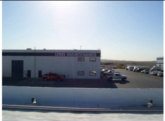
View to East
