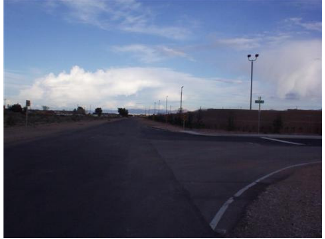
View to East
