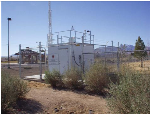
View to South
