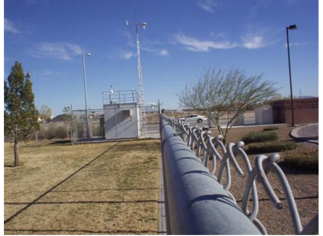
View to East
